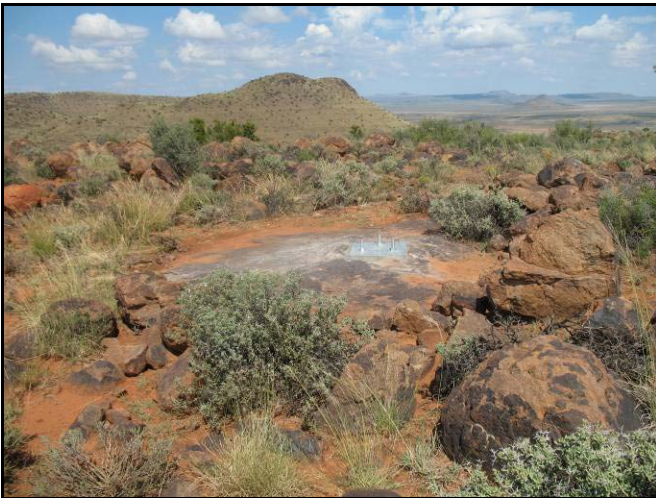
Figure 16 Base of Wind Measuring Mast 3 (temporary). Mast still to be erected
