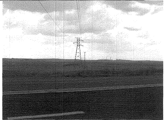
Plate 9: Amajuba Power Station
