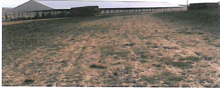
Figure 3. One shed has been constructed. The second will be constructed from the position of this photograph.
