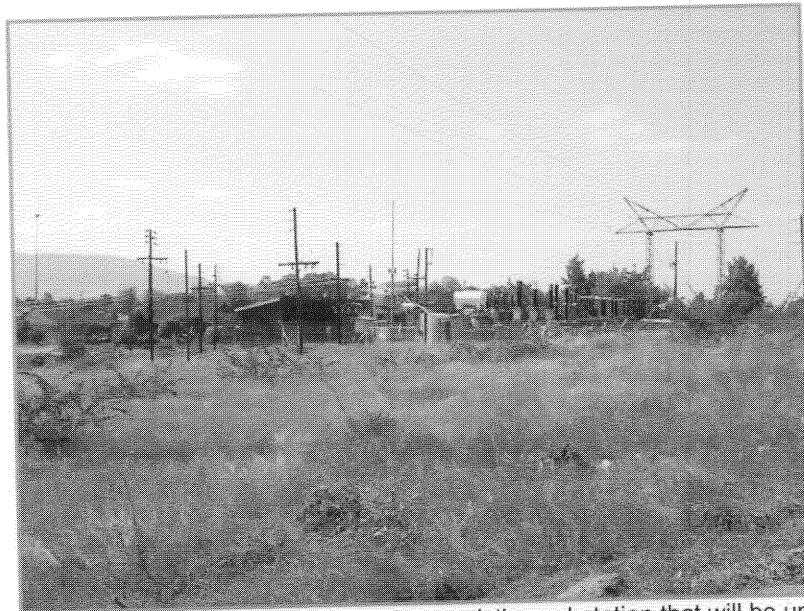
Plate 1: Propose Matsulu Substation site. There is an existing substation that will be upgraded to suite the new capacity.
