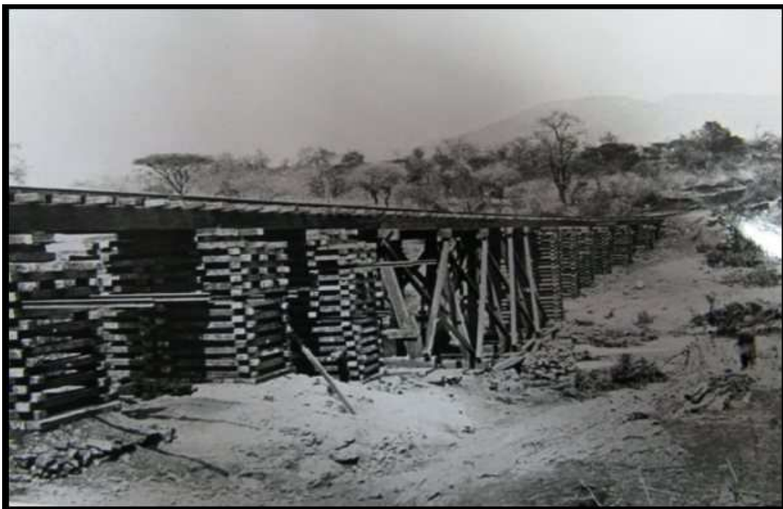
Fig. 4.5. Kaapmuiden bridge constructed by the Six Companies of the Brigade of Guards in two days during the ABO, c. 1899-1902.
