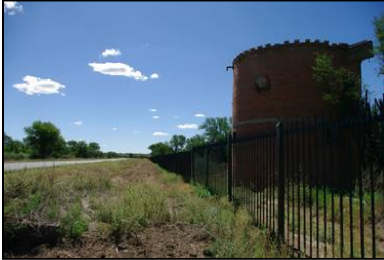
Figure 9: View of a structure post dating 60 years of age situated in immediate proximity to the western part of the road reserve study site where the pipeline has already been closed
