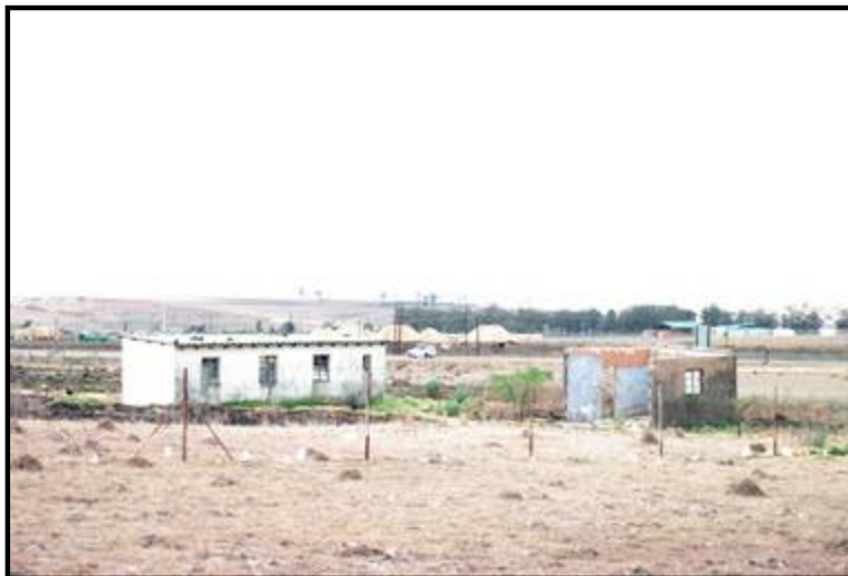
Figure 12: View of the C2.2 farming infrastructure structures, fenced within the school yard
