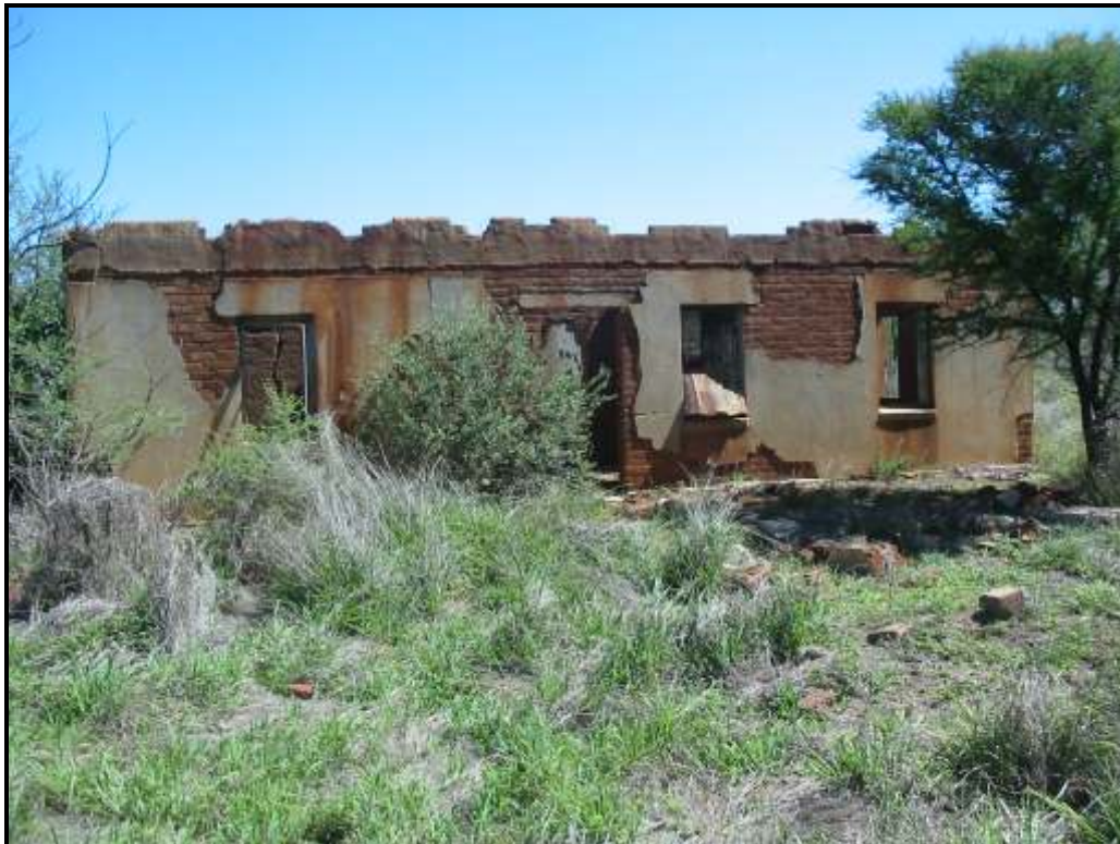
Figure 1: Ruin viewed from the south
