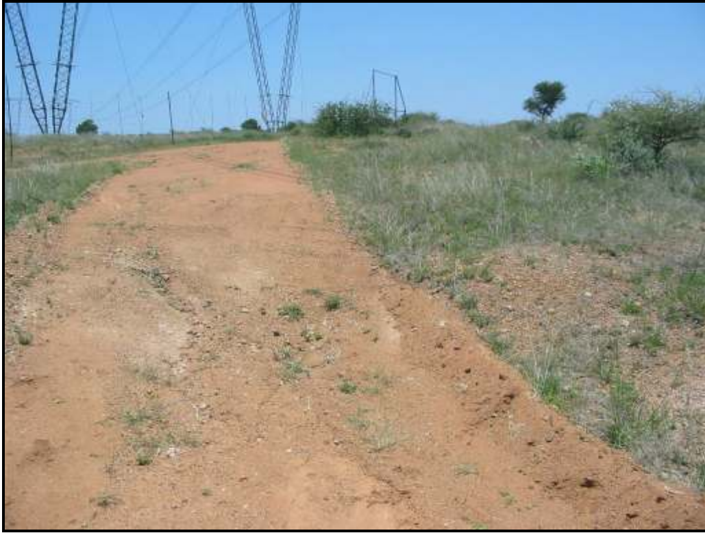
Figure 12: General Site conditions
