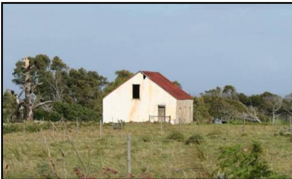
FIG. 8: OLD FARM BUILDING
