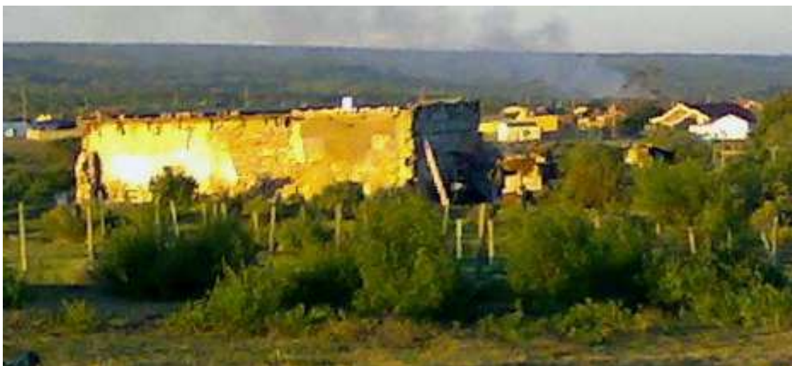
Figure 4. The rectangular farm building on the property, F in Fig.3.
