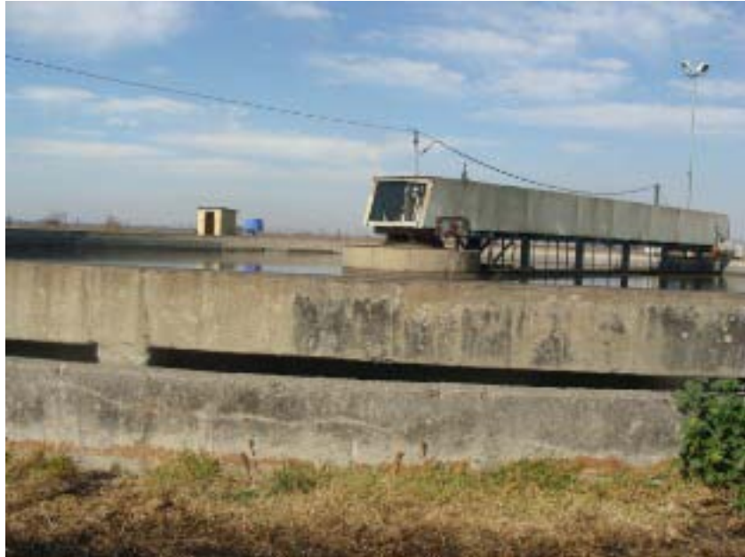
Figure 5: Photograph of existing dam.
