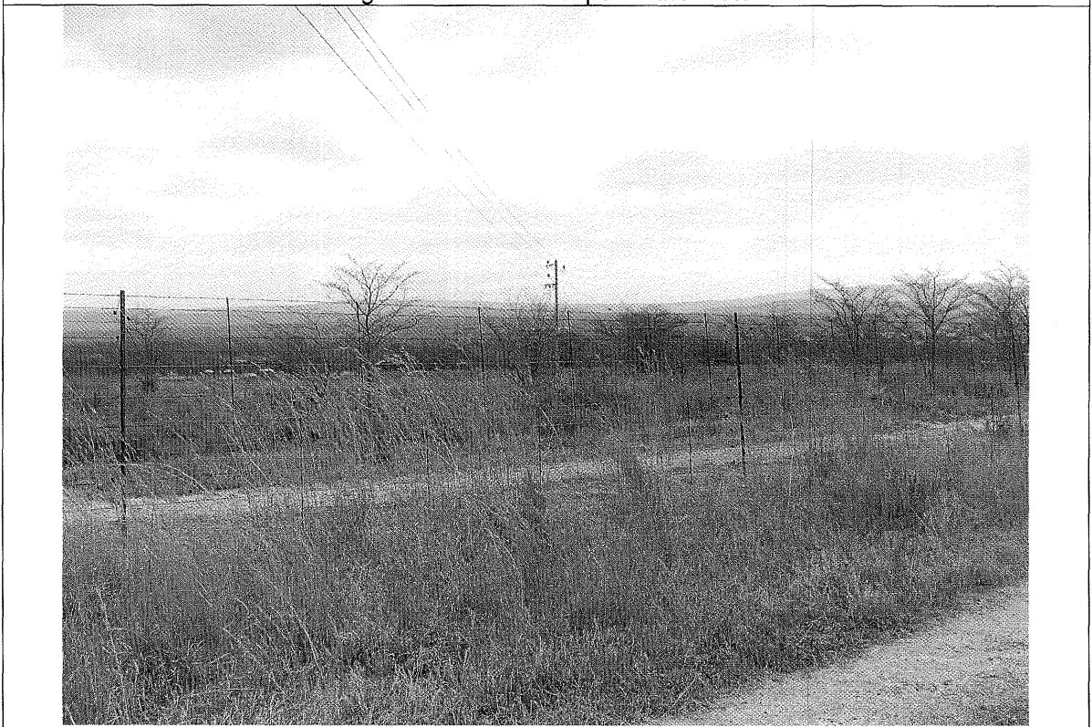
Fig. 8 General view of powerline route
