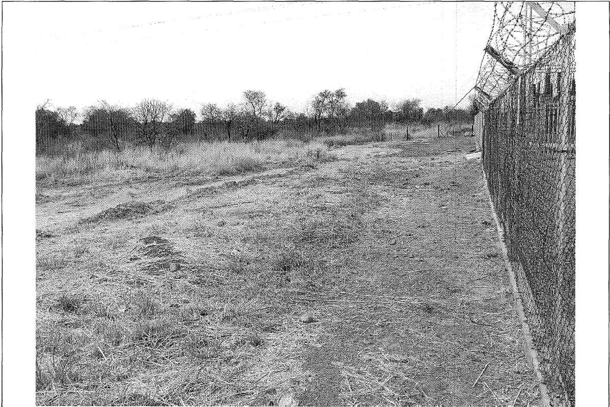
Fig. 1 View of sub-station site 1
