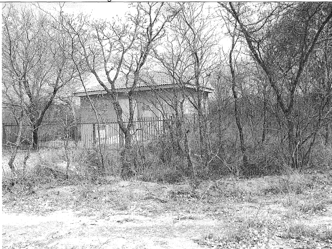
Fig. 6 View of new sub-station site 3
