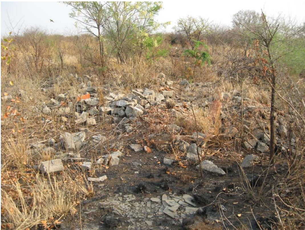
Photo 4: View of some of the illegal dumping on the site.
