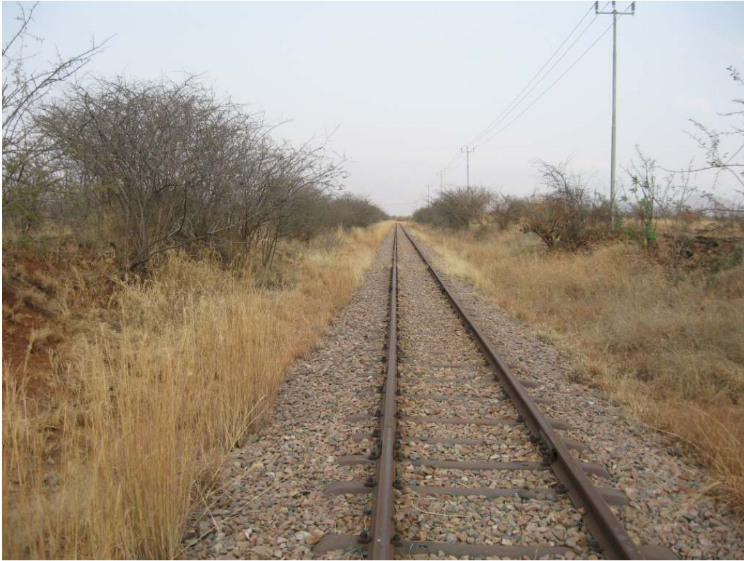
Photo 3: View of the railway line on the northern side.
