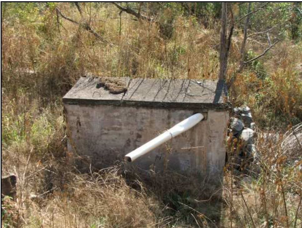
Fig. 5. Site 3. Water pump enclosure.
