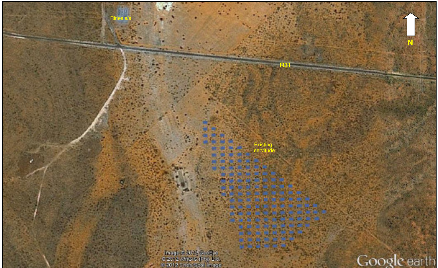
Figure 3. Aerial photographing illustrating the proposed layout of the CPV panels for the Mount Roper Solar Energy Plant
