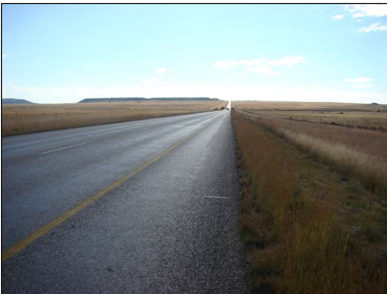
Fig.4 N1 Section 14, 81,6km.
