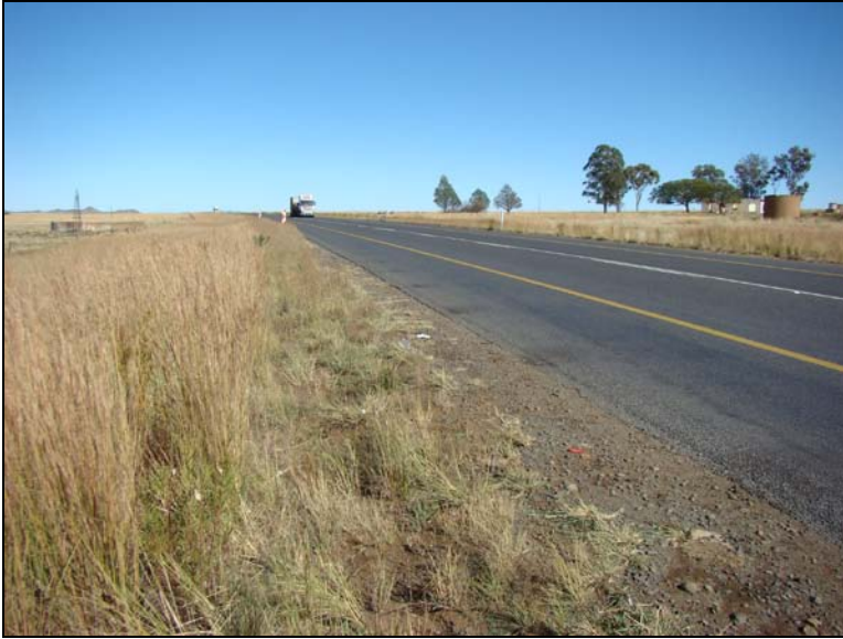
Fig.21 N1 Section 14, 42,4 km.
