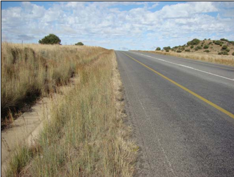
Fig.3 N1 Section 14, 85,0km.
