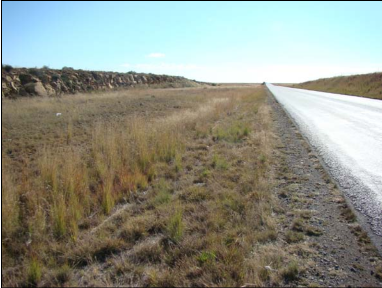
Fig.1 N1 Section 14, 90,0km.
