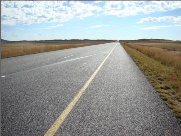
Fig.13 N1 Section 14, 61,9 (62,0) km.
