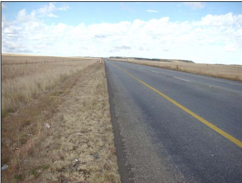
Fig.2 N1 Section 14, 88,4km.
