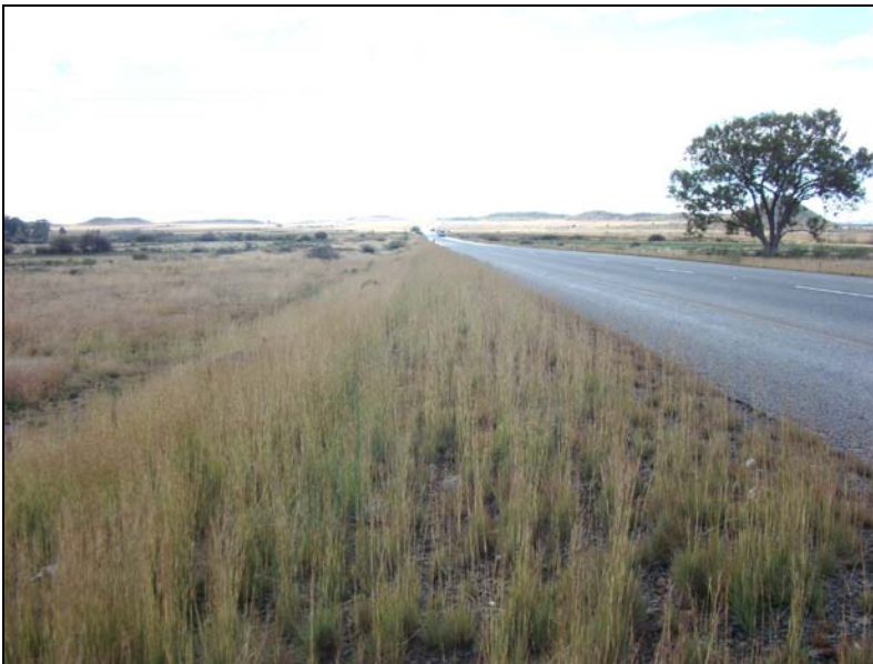
Fig.12 N1 Section 14, 65,2km.
