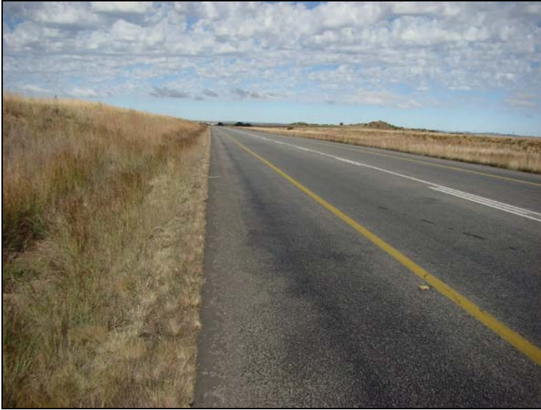
Fig.5 N1 Section 14, 79,4km.
