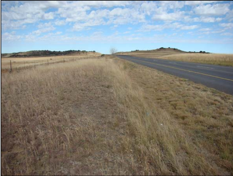
Fig.7 N1 Section 14, .69,6 km.
