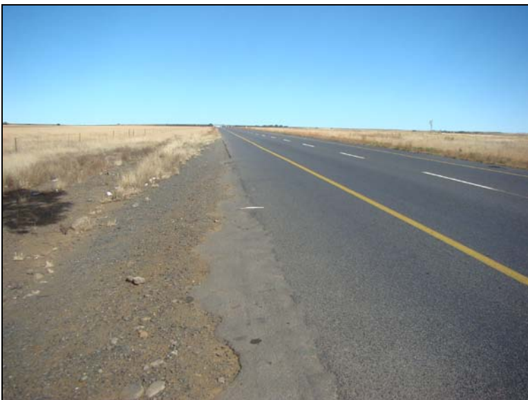
Fig.20 N1 Section 14, 50,4 (50,3) km.
