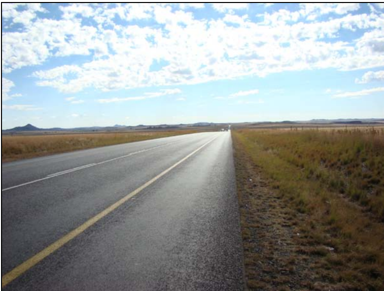
Fig.14 N1 Section 14, 60,3 (60,4) km.
