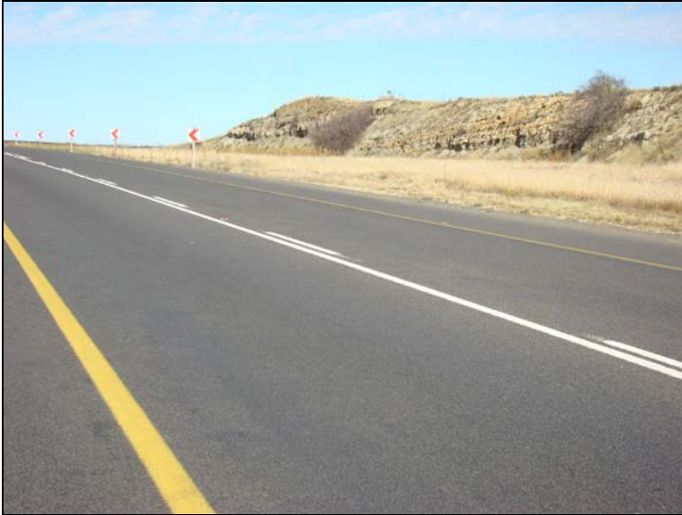
Fig.11 N1 Section 14, 64,25 km.
