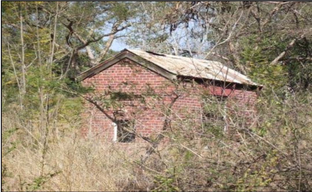
Fig. 12. Site N4 9/7. The old Pump Station or building at Krokodilpoort Station.
