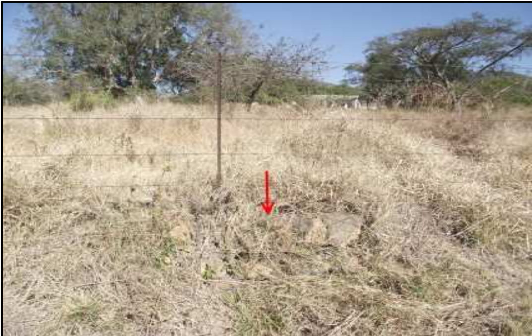
Fig. 14. Site N4 9/9. The section of wall which may be associated with Poort City.
