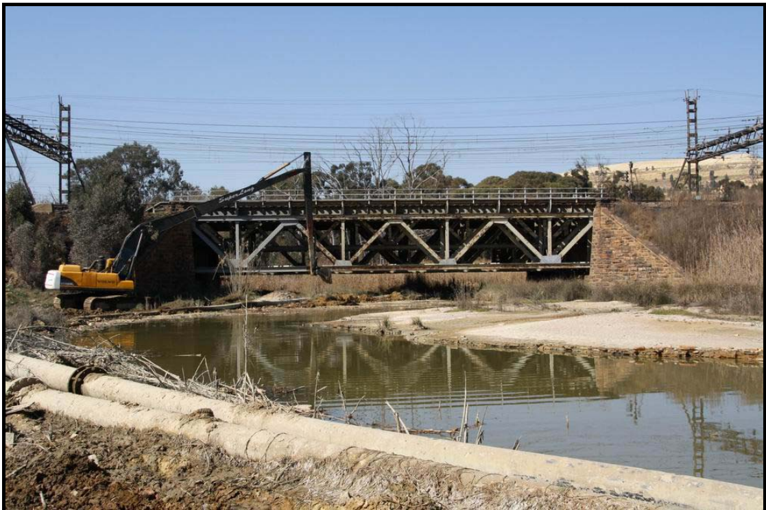
Fig. 3. The old train bridge.
