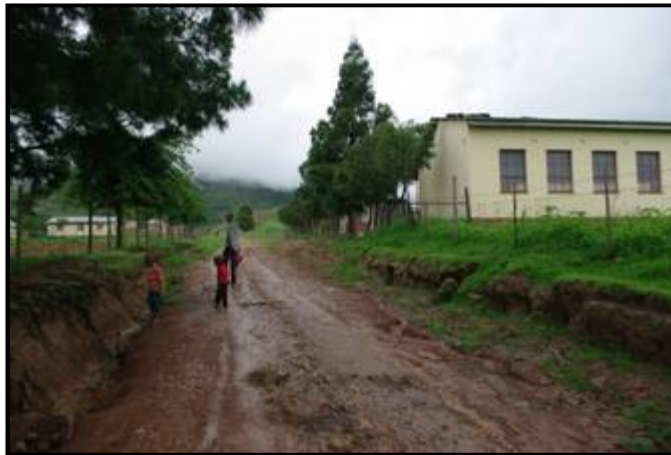
Figure 17: Well defined development corridors throughout Lower Gqaga – D (vicinity of SP71)
