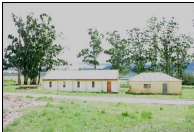
Figure 38: From left to right – Iron Age tradition hut ruins, the contemporary church and the Colonial Period (early 1900's) mission church
