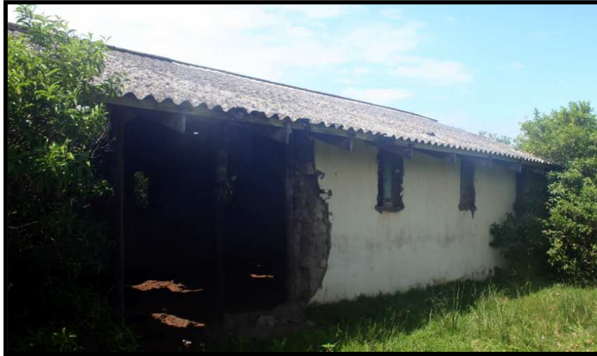
FIG. 3: VIEWS OF HISTORICAL BUILDING AT NKA01
