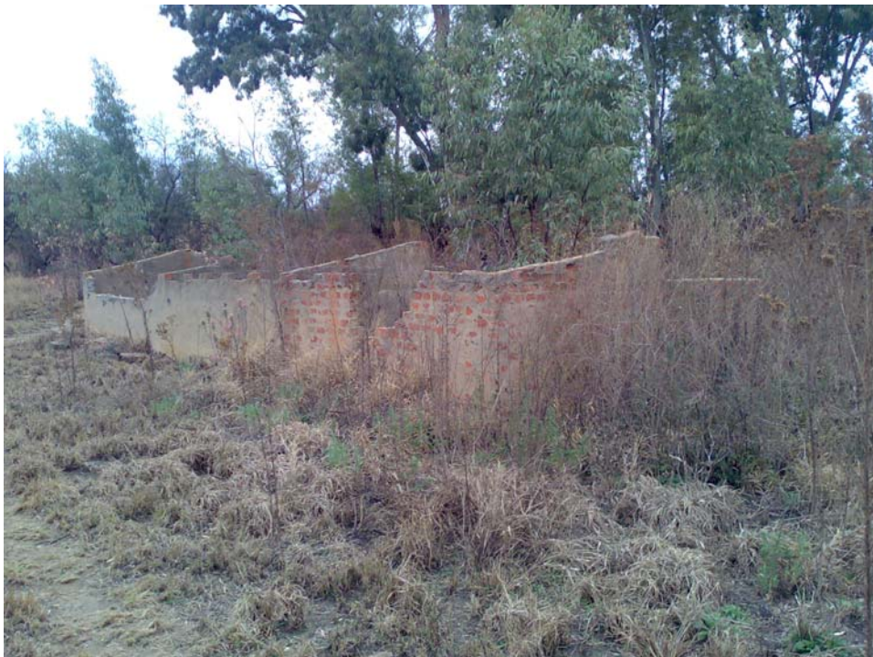
Figure 6: Remains of structure for livestock.
