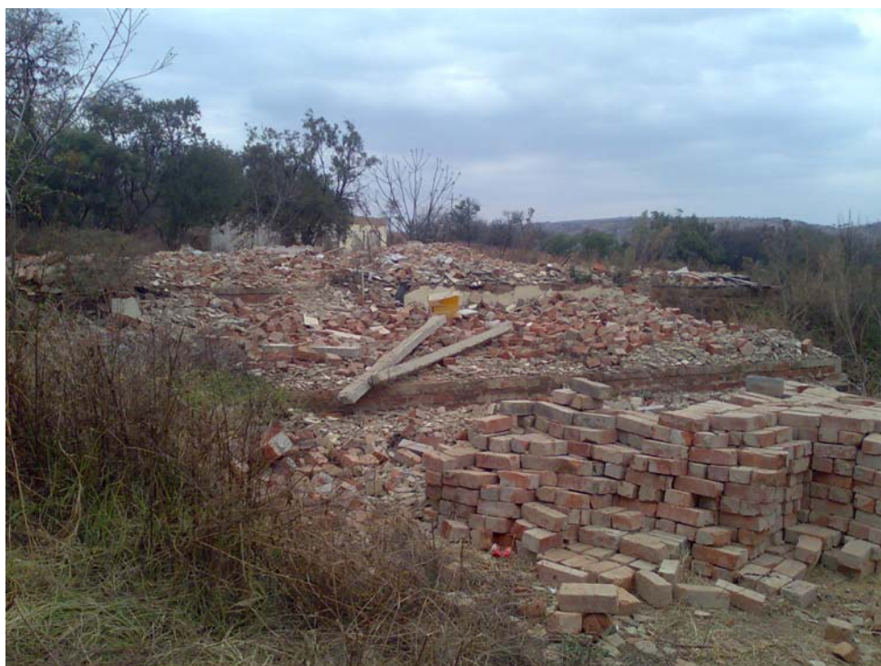
Figure 4: Remains of demolished house.
