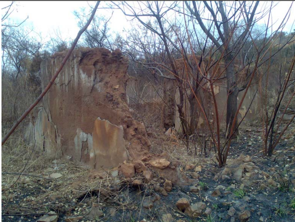
Figure 3: Remains of demolished house.
