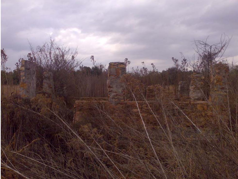
Figure 5: Remains of structure for livestock .
