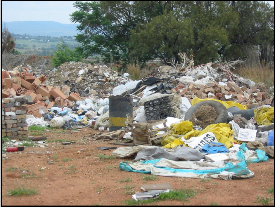
• Figure 4: Dumping on site
