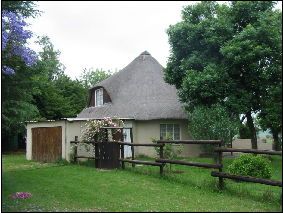
• Figure 2: Modern dwelling on site
