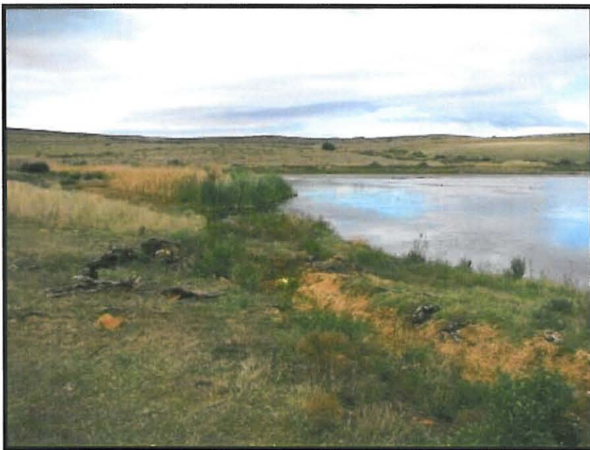
Figure 4. View of the Jan Harmsgat Dam facing north west
