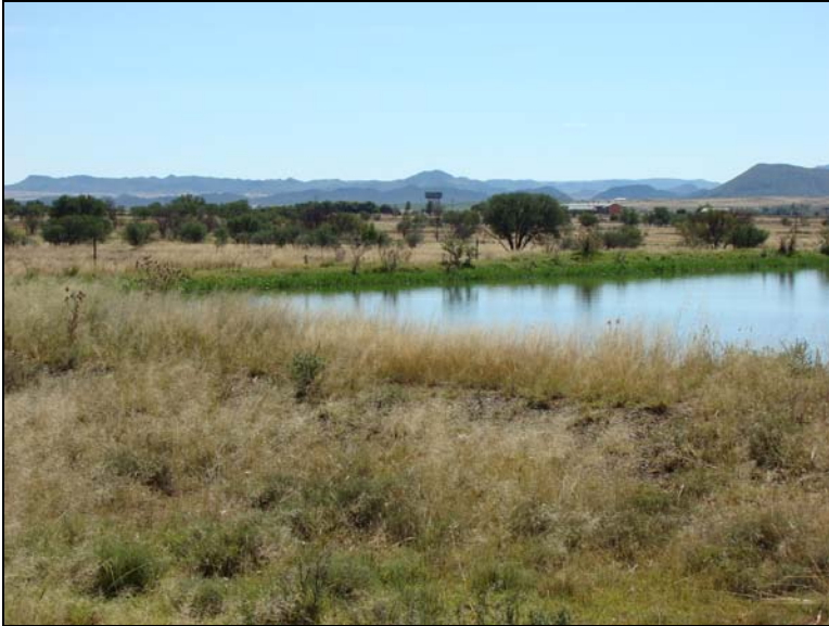
Fig.2 View from across the existing sewer dams facing east.
