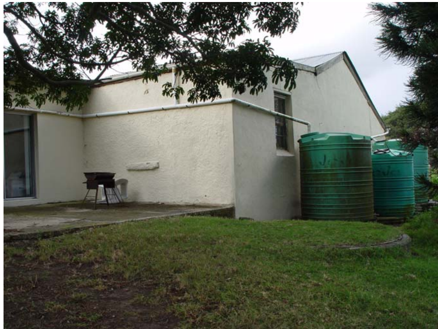
Figure 11: Veranda and back of house.
