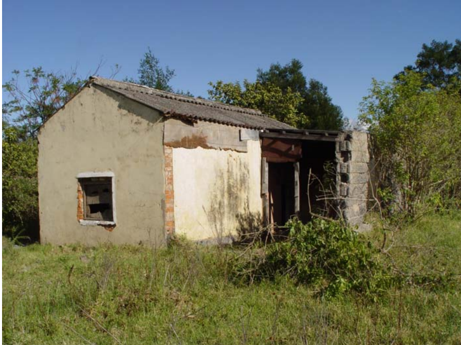
Figure 4: Dilapidated old house.
