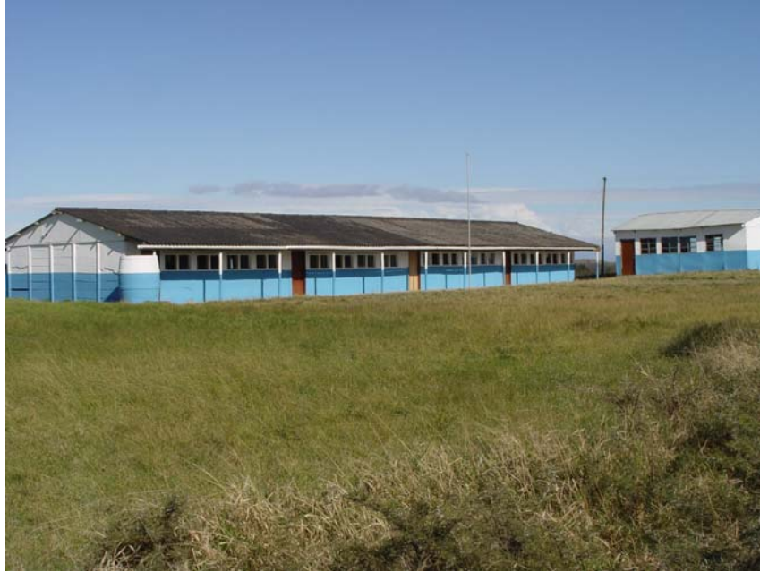
Figure 5: Local school building.
