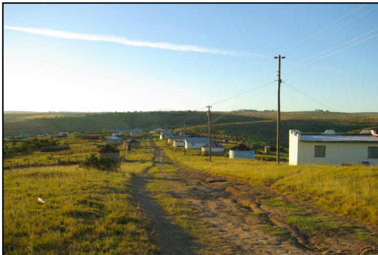
Figure 9: View of the existing road portion through Nyathyora Village
