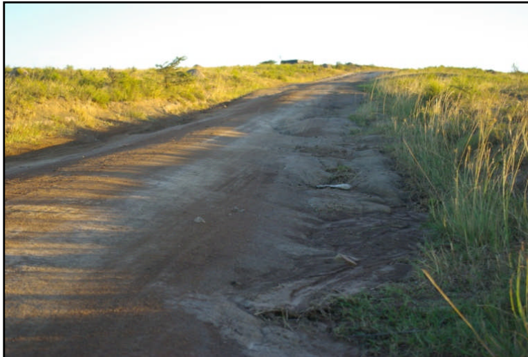
Figure 8: General view of the Nyathyora internal roads study site - Nyathyora area
