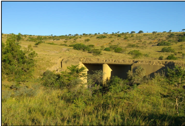
Figure 6: View of the bridge south of Mtwaku Village
