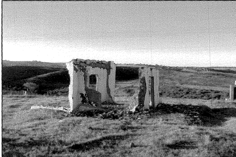
Figure 10: Structure ruins in Nyathyora village post dating 60 years of age
