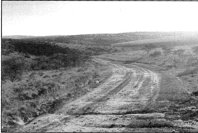
Figure 7: General view of the Nyathyora internal roads study site - Mtwaku area
