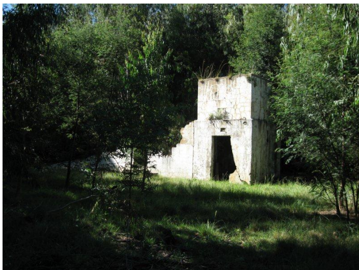
Figure 5. OB 1 Remains of an old farm house.
