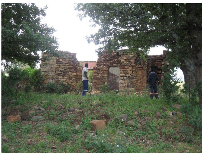
Figure 38. OB 16 Remains of old farm house and associated buildings.
