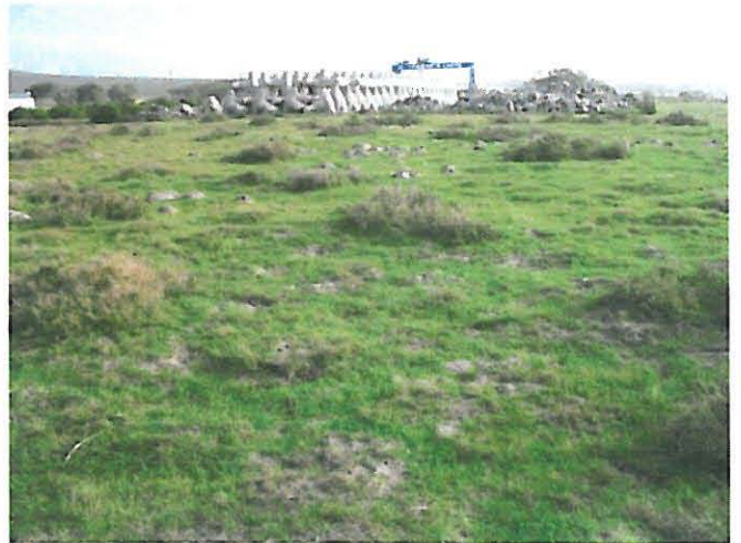
Figure 12. View of the site facing west
