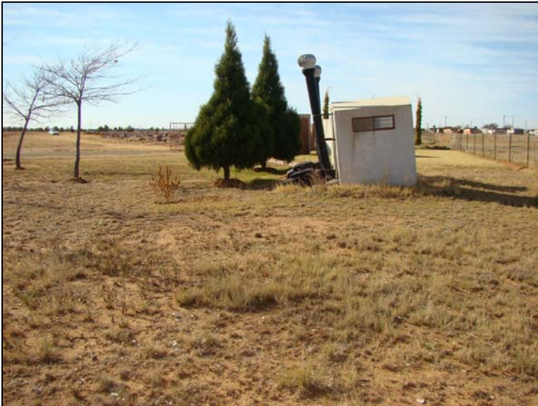
Fig.7 Ablution facilities near the entrance to the Pumlani Cemetery at Thabong, Welkom.
