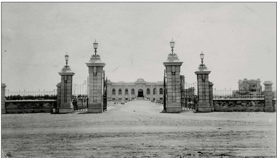
Figure 12 - Historic photograph depicting the front entrance gates of the Vereeniging Pumping Station which were completed during August 1923. The Engine Room (centre) and Offices (right) can be seen behind the gates and fence (Museum Africa, Images Collection, PH2007-14433).
