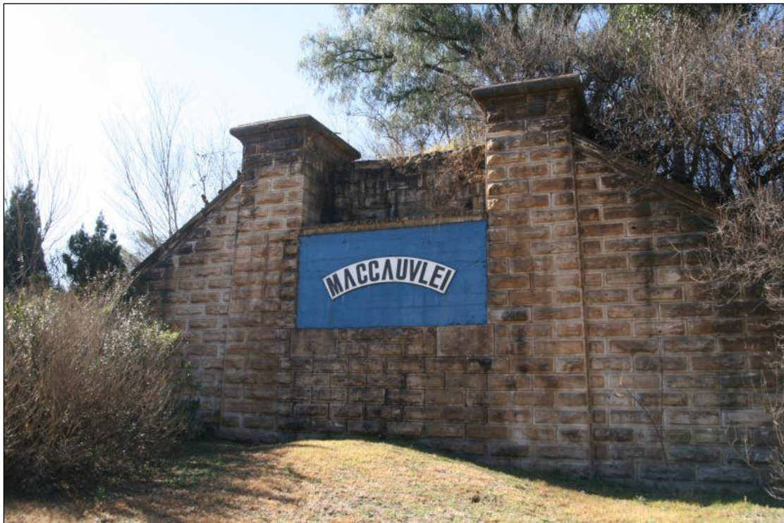
Figure 6 – Old bridge foundation close to where proposed crossing to the Gauteng Province over the Vaal is (Site RW1)
