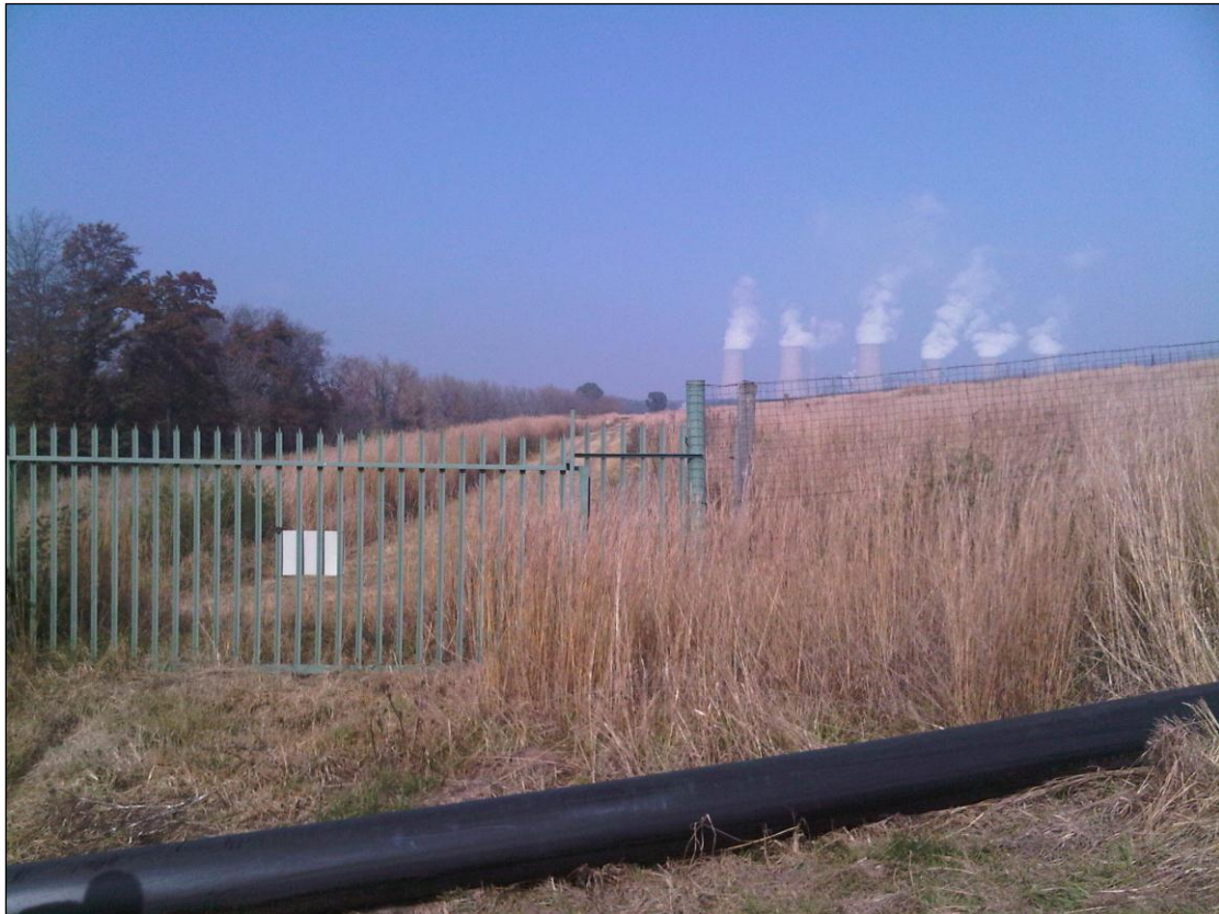
Figure 3 – View of servitude toward Lethabo pump station (Taken right across the river from the Suikerbos Pump station)
