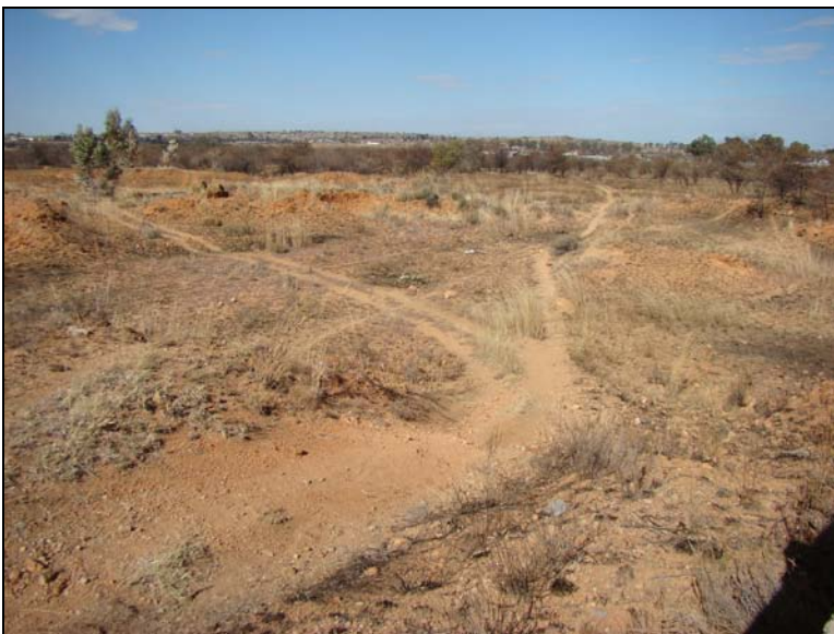
Fig.10 Point F showing damage to the soils surface.
