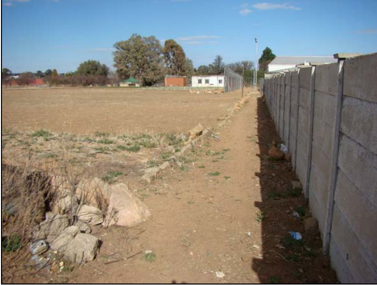
Fig.3 Point C facing south towards the old prison.
