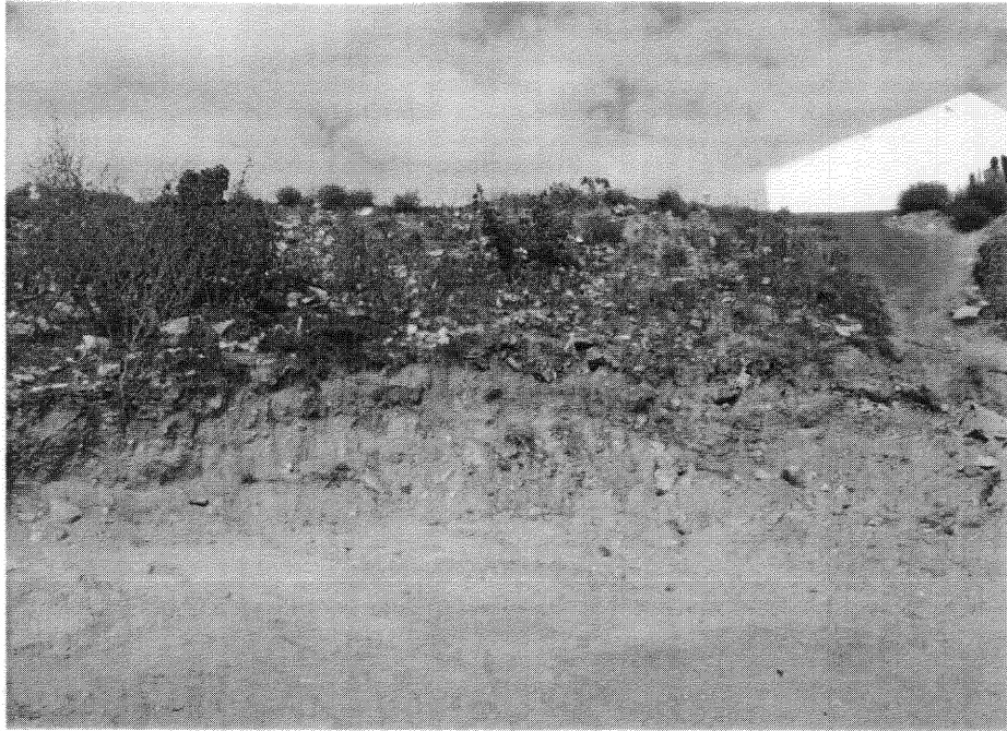
Figure 5: Section of wall showing in situ midden
