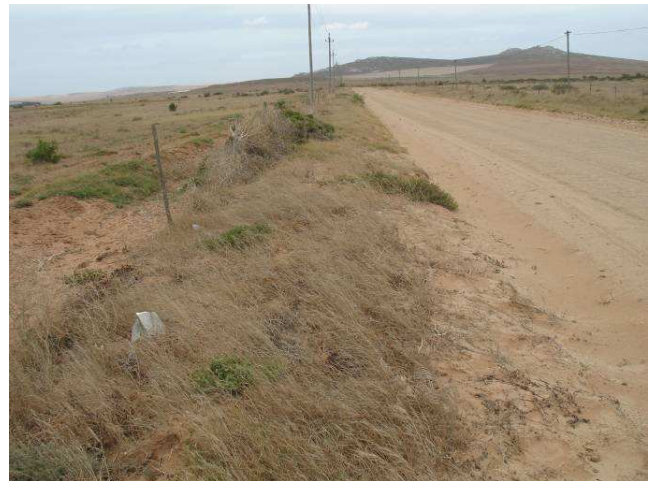
Figure 14. View of pipeline route C facing north
