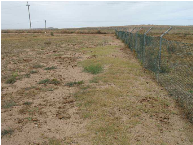
Figure 12. View of pipeline route facing east
