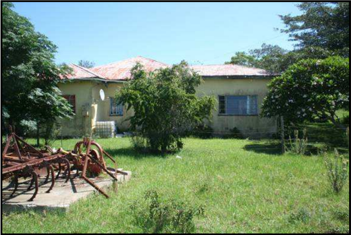
FIG. 5: FARM HOUSE AT PGE05
