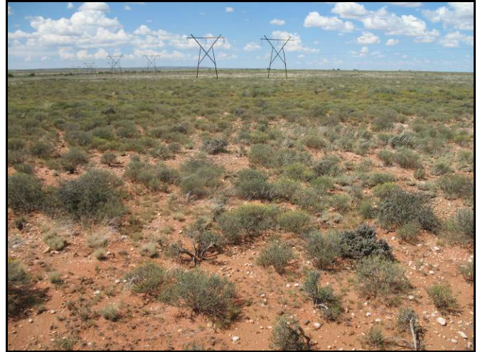
Figure 9. Copperton PV site view facing north west
