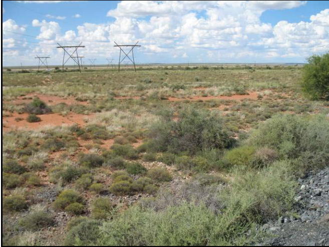
Figure 12. Copperton PV site view facing north east
