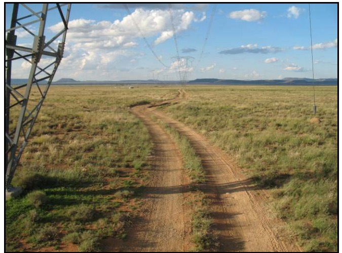
Figure 20. South East Option access road facing north
