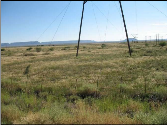
Figure 11. North West Option powerline servitude facing east
