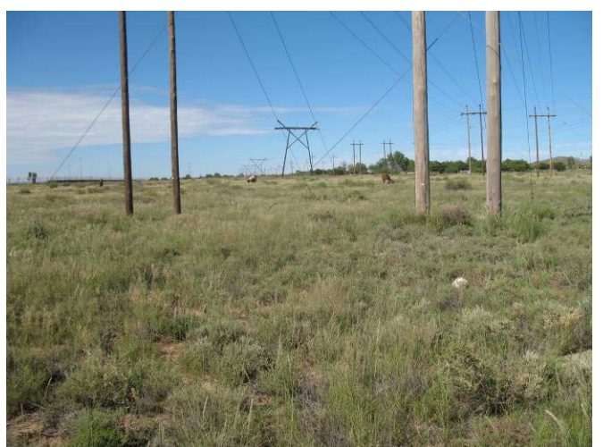
Figure 10. North West Option powerline servitude facing west toward De Aar
