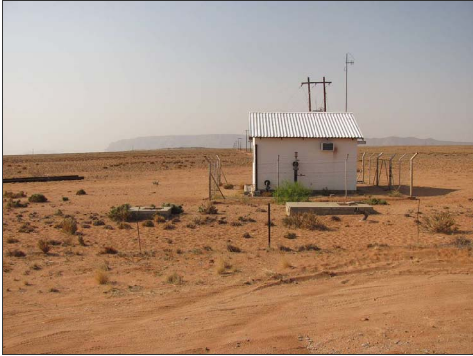
Existing infrastructure at the eastern end of the pipeline
