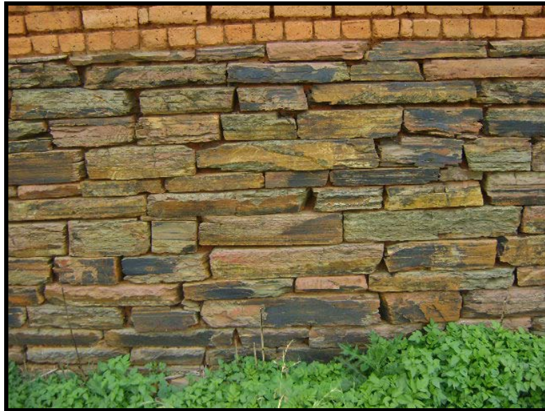
Detail of slate in an old building in Machadodorp
