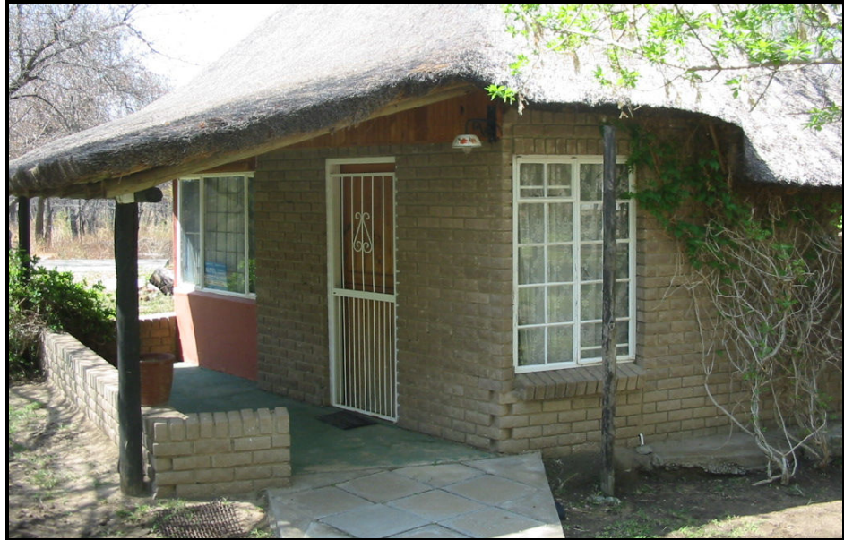
•Figure 2: Structures on site
