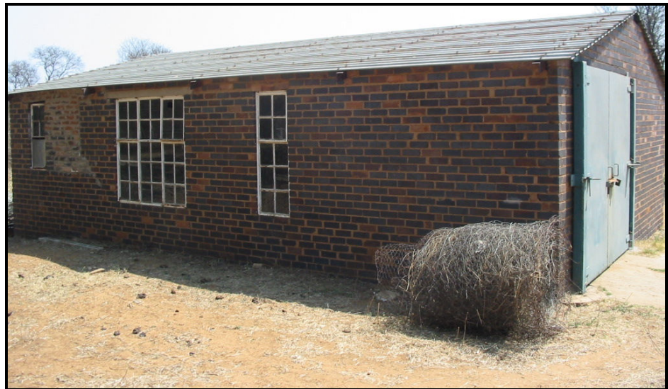
• Figure 1: Modern building on site
