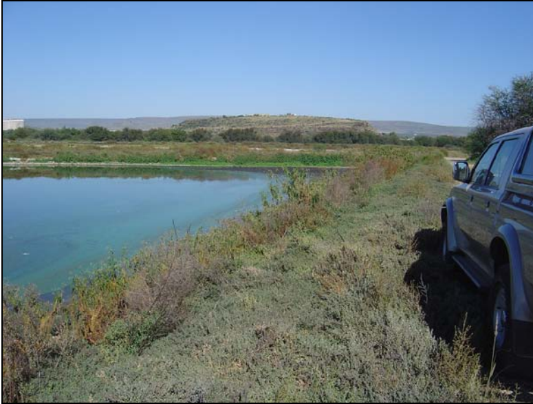
Fig.1 Existing sewerage oxidation dams at Prieska, Northern Cape.
