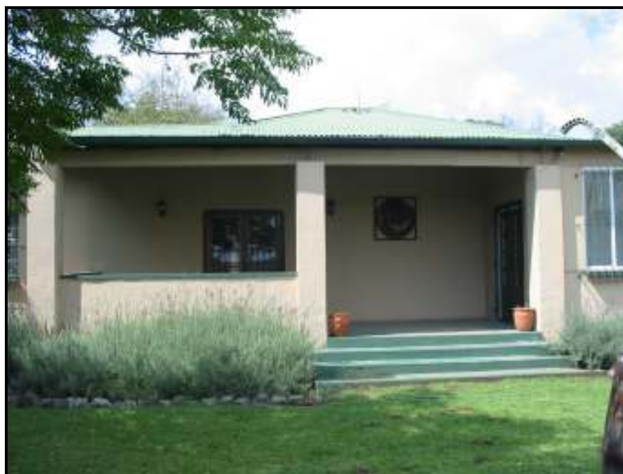
Figure 4: Historical dwelling nr1 viewed from the west
