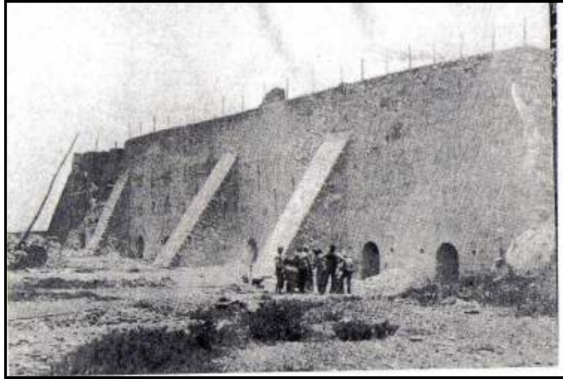
Figure 1: A 1907 photograph of the kilns of the Irene Lime works.
