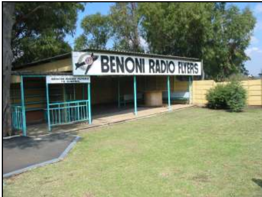
• Figure 1: Modern structure on site
