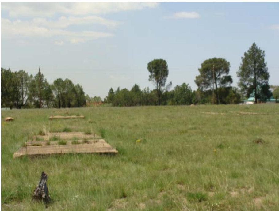
Figure 5: Concrete foundations at site no 1.
