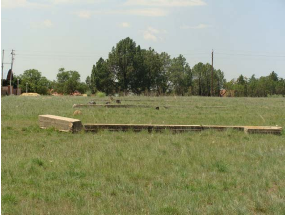
Figure 4: Remains of concrete pillars at site no 1.
