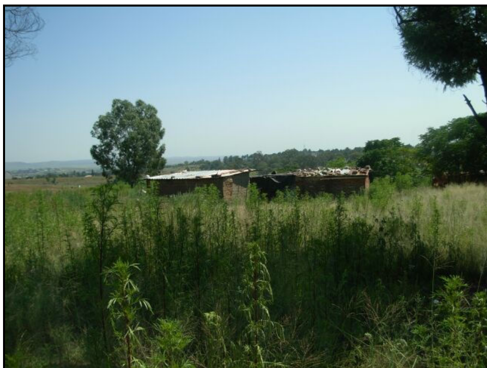
Figure 2: Informal housing on site
