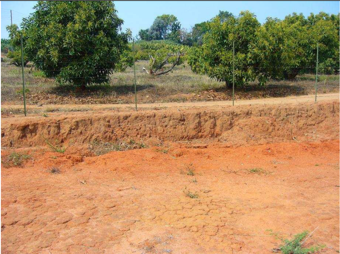
Fig 3. View of boundary fence where soil was removed and slag etc. was noted in the profile.
