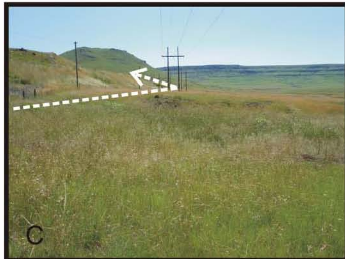
Figure 3. Section 1, looking north. Arrow indicates layout of pipeline (A&C). Exposed mudstones of Tarkastad Subgroup (B).
