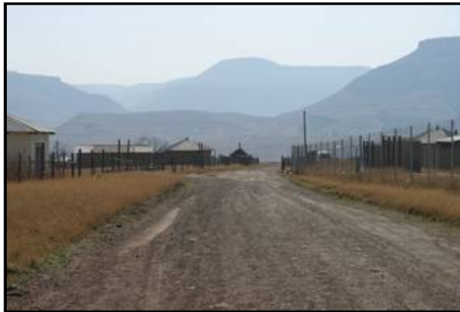
Figure 11: View of the line route development area through Mareleni Village - 2
