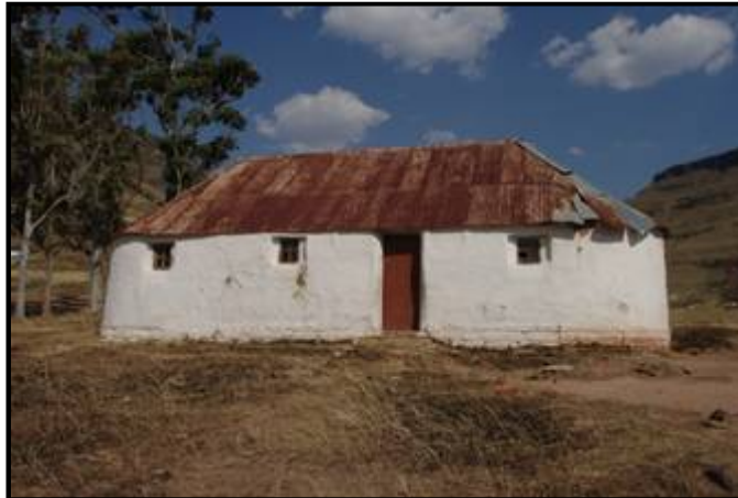
Figure 53: Close-up of the Site H9 structure
