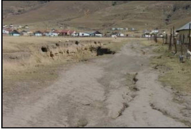
Figure 13: View of the line route study site – Sidindi Village
