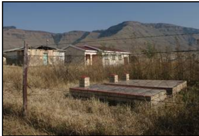
Figure 46: General view of Site C5
