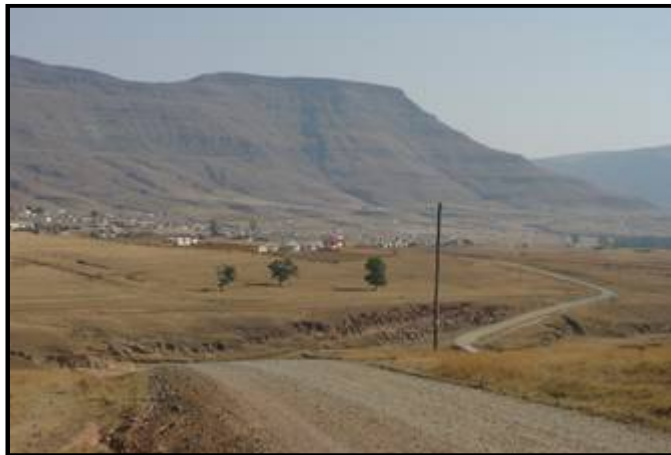
Figure 12: View of the line route along the main access road (Mareleni Village)
