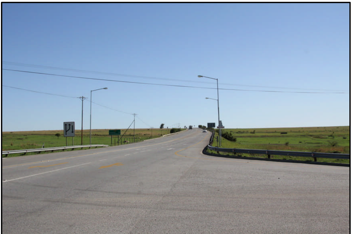
Fig. 9. Looking north over the N1.
